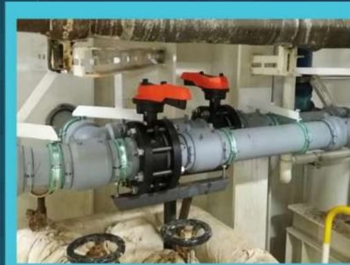
Replacement of the Cunipress Savinox black water system to G.F fuseal PP System
