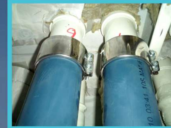
Replacement of the Cunipress Savinox black water system to G.F fuseal PP System
