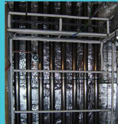
Replacement of the steckdrain piping black or grey water system to Coes Blue Power system
