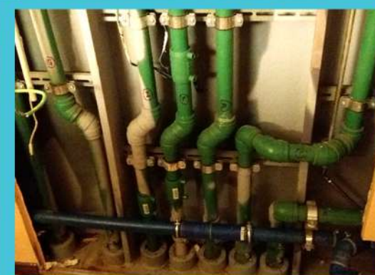
Replacement of Coes piping system to G.F piping system
